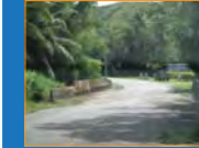
Benny Espinosa Avenue, Merizo - Old bridge with erosion problems.
