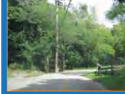
Chalan Jesus R. Quinene, Merizo - Utility pole in clear zone.
