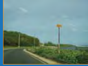
Route 4, Merizo - Missing and old signs.
