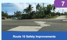
Route 10 Safety Improvements
