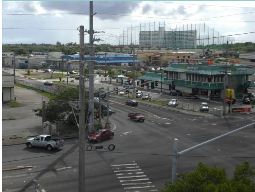
Figure 5-11: Hamburger Highway (Route 27a)—Before
