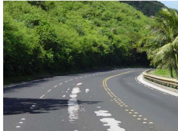
Figure 3-12: Sample Deteriorated Pavement Conditions
