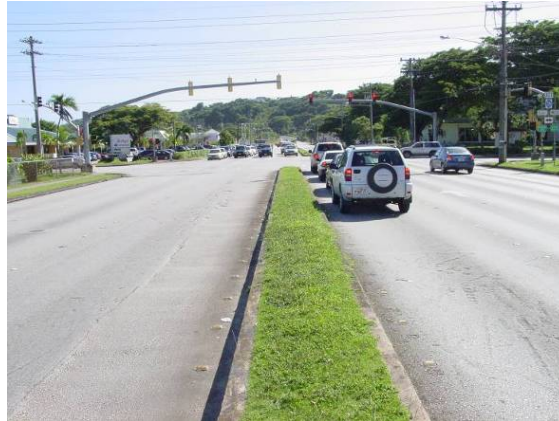
Figure 3-13: Sample Traffic Signal
